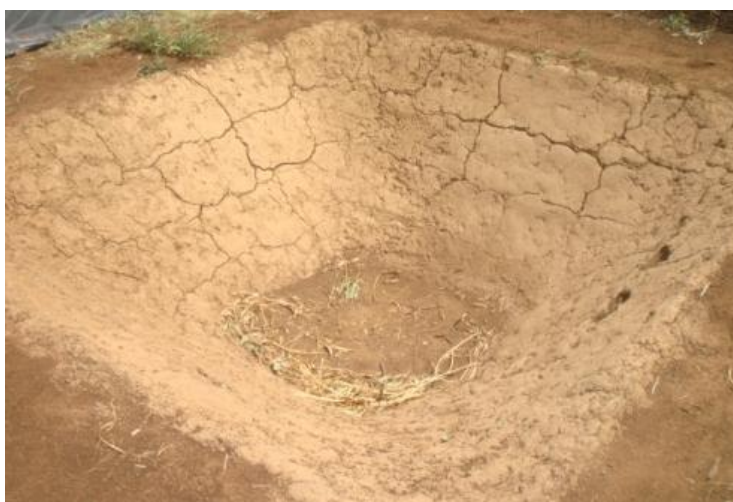
Figure 8. Actual shape of cement + soil lined pond
